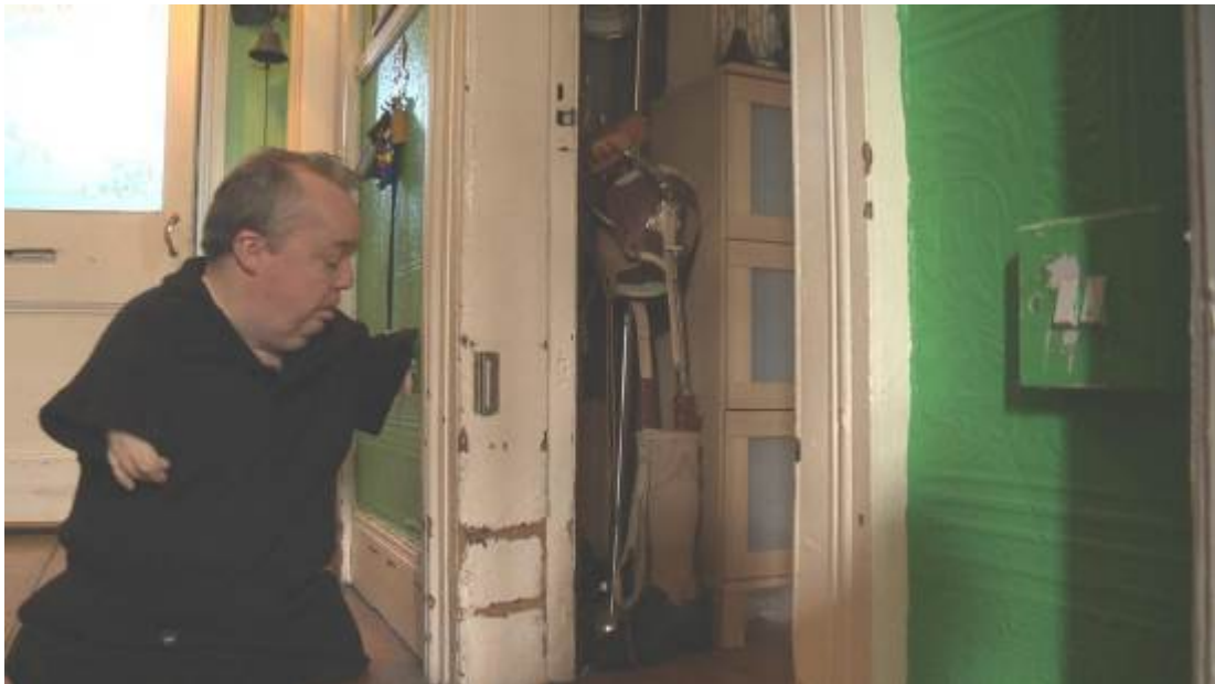
Figure 6 - Electric light switches installed at a low reachable level. Note the door has been removed to accommodate a wheelchair, and shows the damage a wheelchair causes to paintwork – requiring extra and costly maintenance
