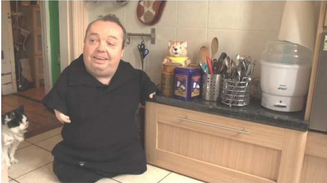
Figure 5 - A thalidomider with no legs and short arms shows his floor-level kitchen units. His kitchen is split between floor-level and normal height units and functions, although it is too small to provide full double functionality. He acknowledges that he and his family need to move to a larger house to provide the flexibility and space for his needs
